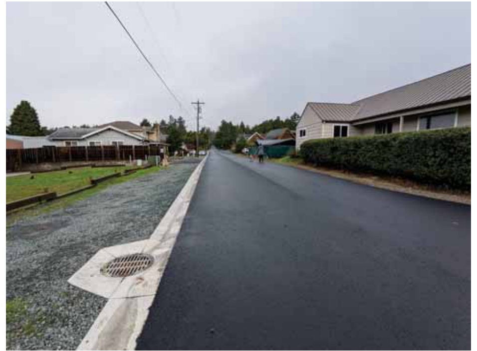
Newly paved local street with stormwater gutter
