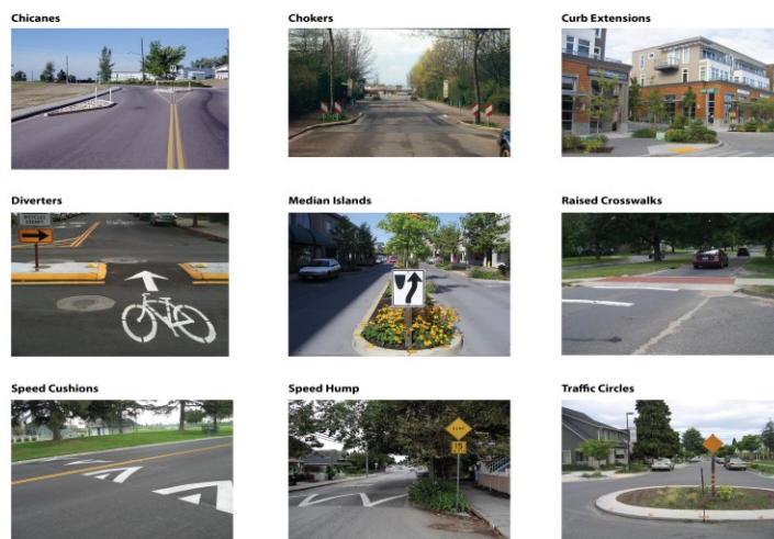
Figure 2 - Nine examples of traffic calming measures for select neighborhood streets.
