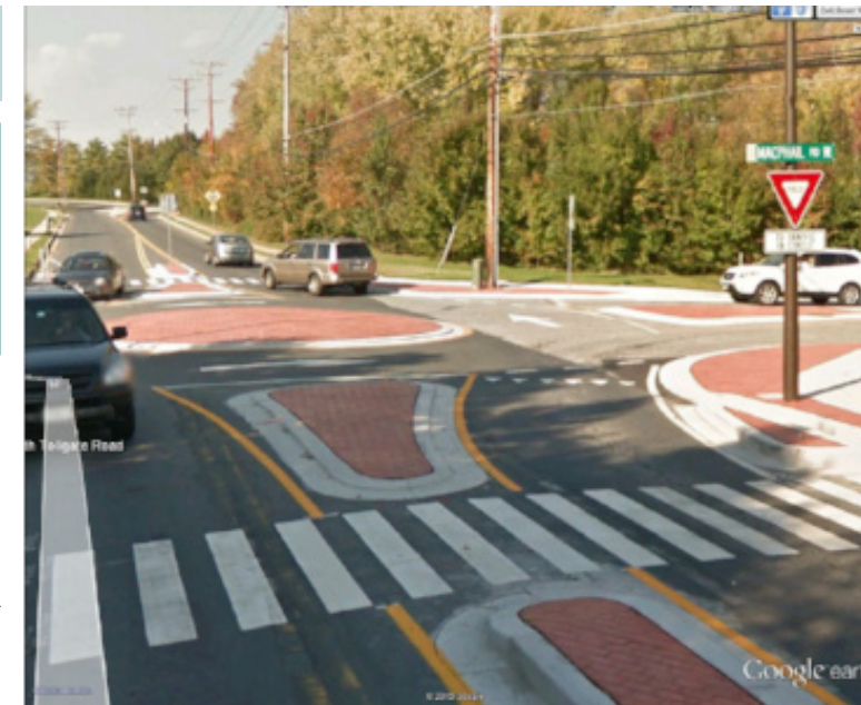
Example of a mini-roundabout with a traversable center island designed for trucks to drive over. Photo Source: Transportation Research Board
