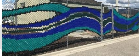
Enhance Existing Chain-link Fences: A low-cost way to brighten up utilitarian barriers.
