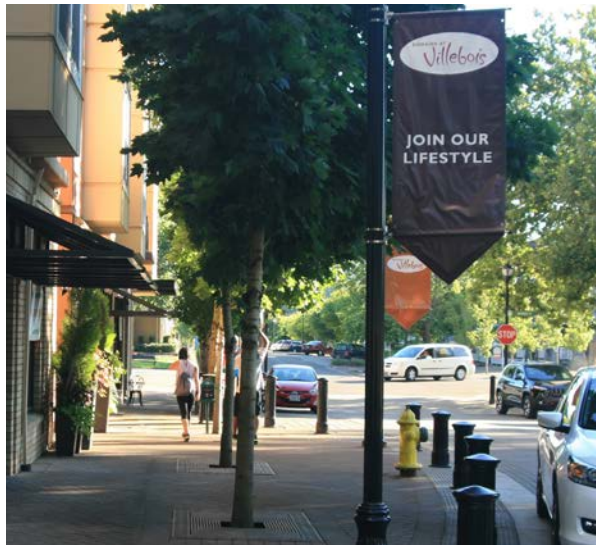
Villebois' main street employs a curbsless street design where the plaza and the street blend seamlessly and bollards, not curbs, mark off the area for cars.
