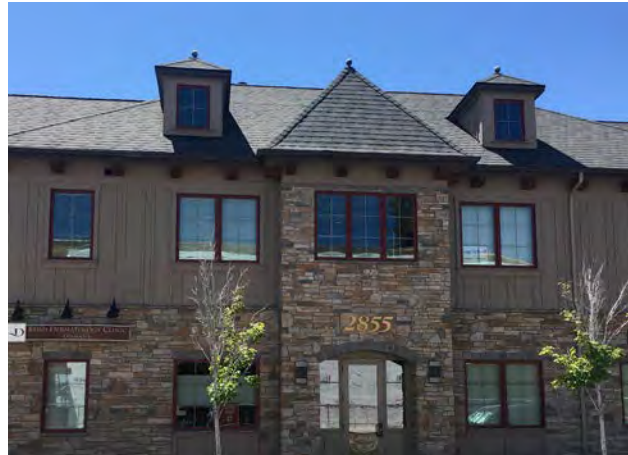
Employment uses adjacent to the town center have attracted a range of tenants including anchor tenants such as HydroFlask.
